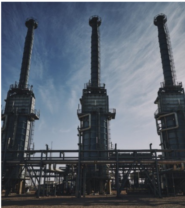
Potential Heat recovery from turbines to replace fuel for heaters
