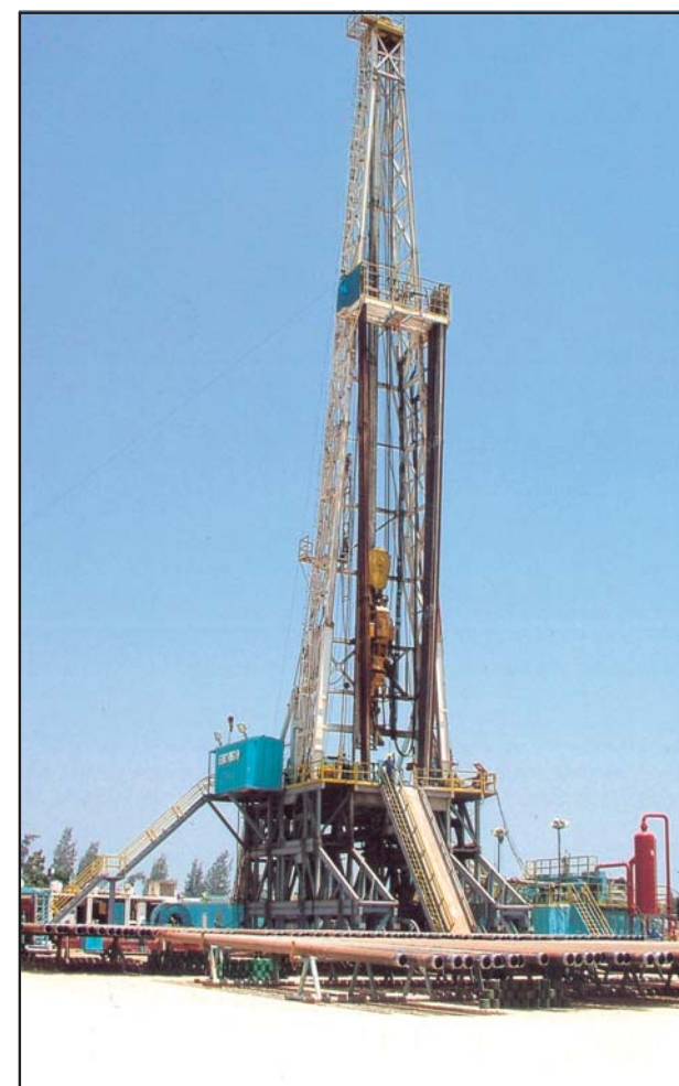
ECDC's rigs have been used in many projects in Saudi Arabia
