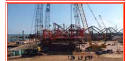
CELLAR DECK LIFTING
